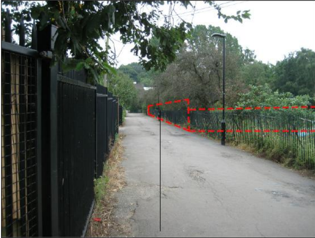
Photo 1: Eastern boundary of site next to public footpath. New chain link fence set behind existing boundary fence
